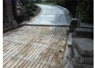
**Sand Bed Paver Overview:** The heating cable may be secured in place by landscape stakes and plastic wire ties, welded wire fabric and plastic wire ties or tape. Do not compress or strain the cable, run heavy machinery, equipment, or vehicles over it. Be careful to avoid stepping on the cold section factory connection of the cable.
