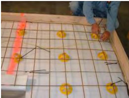
3. Attach Tuff Cable element to welded wire fabric with wire ties, as shown in the following section, making sure Tuff Cable NEVER crosses through the indicated joint.
