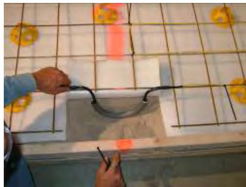
4. Use a Heatizon Tuff Cable Joint/Mark Jumper Kit (Heatizon Part # JUMPERKIT) to extend Tuff Cable through any joint. Note that the Tuff Cable does not cross the indicated joint at any point.
