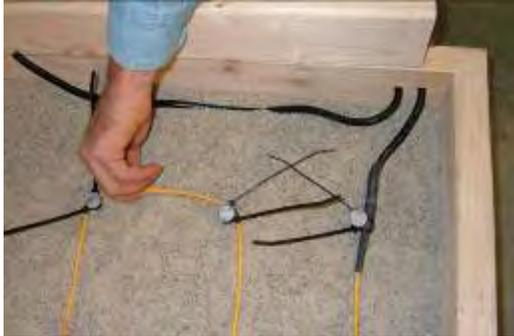
**Step 5.** Connect one Cold Lead to Tuff Cable, then round the spikes with the Tuff Cable at each end and tie the Tuff Cable to the spikes using plastic wire ties. Make a continual loop of the Tuff Cable, making sure the end of the Tuff Cable returns to the Cold Lead location. Leave an extra 12" of Tuff Cable at the start and finish to make eventual connection to the Cold Leads.
