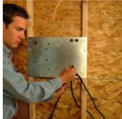
**Note: All Heatizon Systems Transformers require one pair of Cold Leads (except for S202 -- 2X2kVA and S203--2X3kVA Transformers which require two sets of Cold Lead pairs). One of the Cold Leads from any given pair connect to the common tap located at the back of the Transformer and the other Cold Lead connects to one of the voltage taps at the front of the Transformer.**
