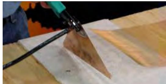
**Step 2: Solder Cold Lead Connection.** Solder all exposed copper strands of Cold Lead with provided solder, heating the butt splice sufficient to draw solder back into the splice.
