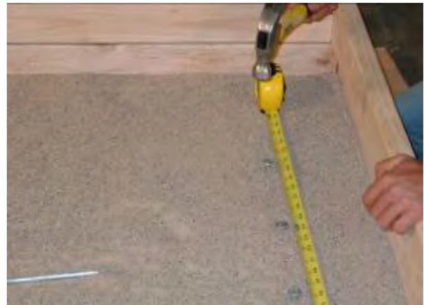
**Step 2.** Create a layout by determining which direction to run the Tuff Cable. Remember that Tuff Cable must be installed in lines that are parallel to one another. Make sure that both the beginning and end of the Tuff Cable element runs are in the same area as the Cold Leads.
