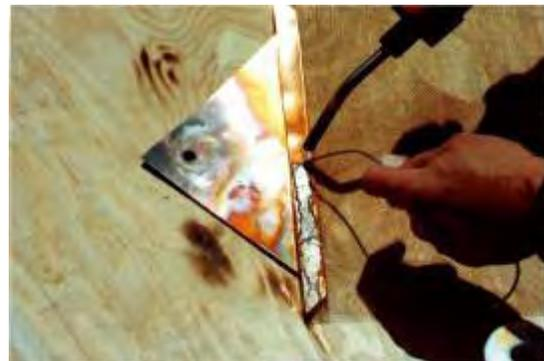
**Step 4: Solder ZMesh connection.** Apply heat to the Transition plate only and never to the ZMesh. Be extremely careful not to burn holes in the ZMesh. Apply the provided solder to the ZMesh. The solder will be drawn back into the fold and create a permanent bond between the Z Mesh and the Transition plate.
