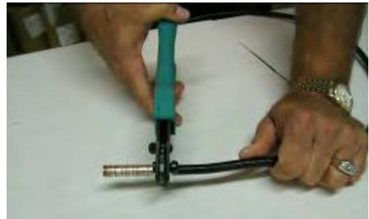
**Step 3: Solder connection.** Solder all exposed copper strands of Cold Lead with the solder provided. Make certain that heat is sufficient to draw solder completely into the splice. Never scorch the insulator on the Cold Lead.
