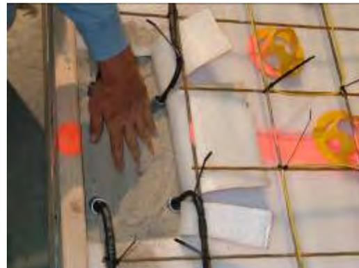
6. Once the jumper is complete, fill in the exposed area with sand so that conduit is completely covered.
