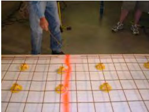
1. After insulation, castle chairs and welded wire fabric have been installed, use spray paint to indicate where any joint (expansion, mark, strike, etc) will be located.
