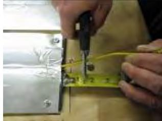
**Step 2: Strip wires.** The Tuff Cable element is connected to the Cold Lead with the Heatizon E210BS90 butt splice connector. This connection is accomplished by stripping back 7/8" of the insulation on the Tuff Cable and Cold Lead wires to be spliced.
