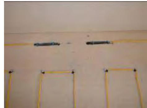
Tuff Cable under hardwood in lightweight concrete.
