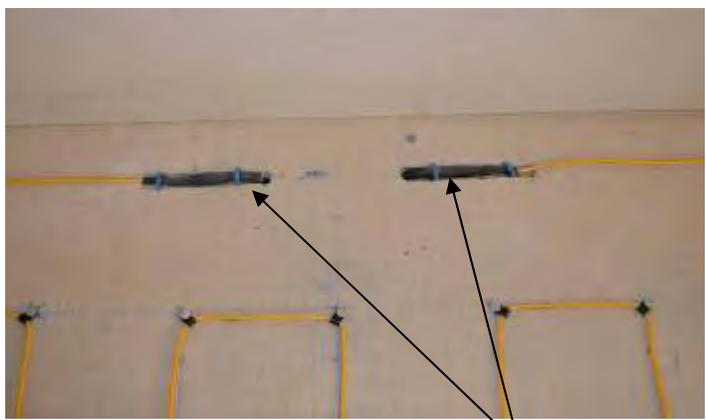
**Note:** All connections between Cold Leads and Tuff Cable must be imbedded in a mortar, asphalt, concrete, Heatizon Heatsink Kit, Invizimelt or other acceptable cementitious heatsink material.
