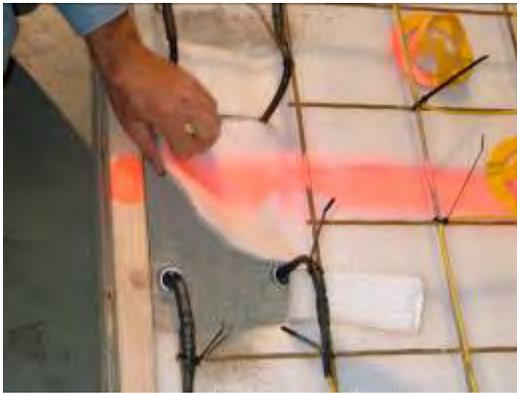
7. Replace the insulation over the top of the sand.
