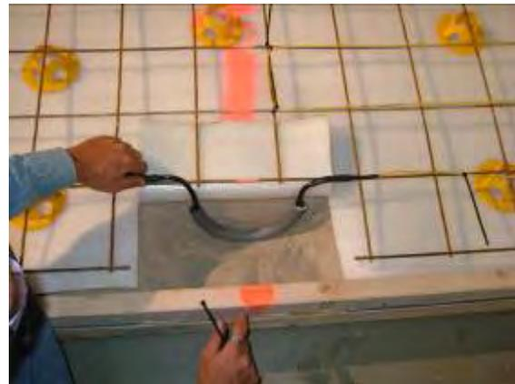
9. If a temperature/moisture sensor such as the M331 or temperature sensor such as the M336 is to be installed in the concrete slab, it must be in place prior to the concrete being poured (See the sensor installation instruction for details).
