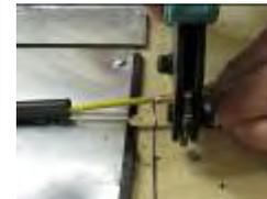
**Step 4: Solder Tuff Cable connection.** Solder all exposed copper strands of Cold Lead and Tuff Cable with the solder provided. Make certain that heat is sufficient to draw solder completely into the splice. Never heat the small end of the E210BS butt splice or scorch the insulator on the Tuff Cable or Cold Lead.
