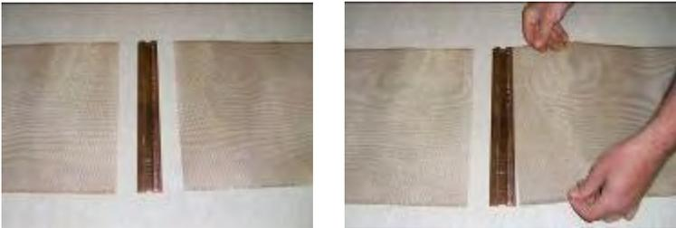
Step 2: Flatten the connection by crimping or compressing the splice plate down on top of both pieces of ZMesh using a short length of 2x4 stud or by tapping gently with a hammer or rubber mallet.
