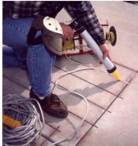
9. Fill all cuts with sealant for asphalt retrofits, or backer rod and sealant for concrete and paver retrofits, in accordance with filler manufacturers recommended procedures.
