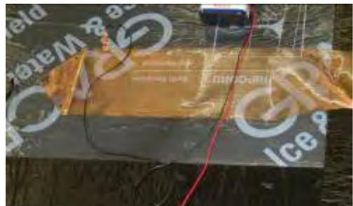
**IMPORTANT! ZMesh must be installed as close to the drip edge as possible in order to reduce the risk of icicle formation.**
