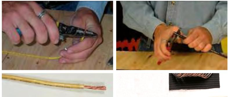
**Step 3: Solder connection.** Solder all exposed copper strands of Tuff Cable and Cold Lead with the solder provided. Make certain that heat is sufficient to draw solder completely into the splice. Never heat the small end of the E210BS butt splice or scorch the insulator on the Tuff Cable or Cold Lead. While connection is cooling carefully slide the sleeve over Tuff Cable end of the E210BS butt splice.
