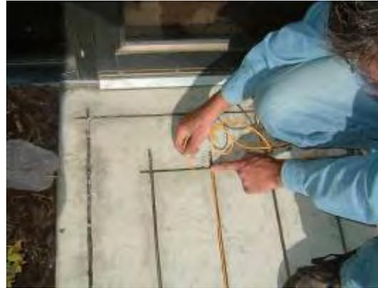
8. The Cold Lead to Tuff Cable element connection is made by following directions in Section 7, "Making the Connection." This connection must be embedded in the concrete, asphalt or pavers.
