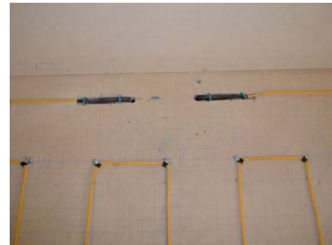
Tuff Cable under tile on a concrete slab
